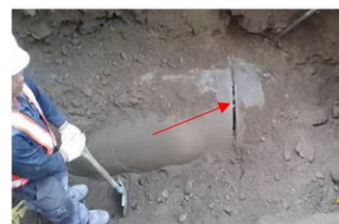
Figure 1. Sinkhole occurrences due to defective sewers [1]
