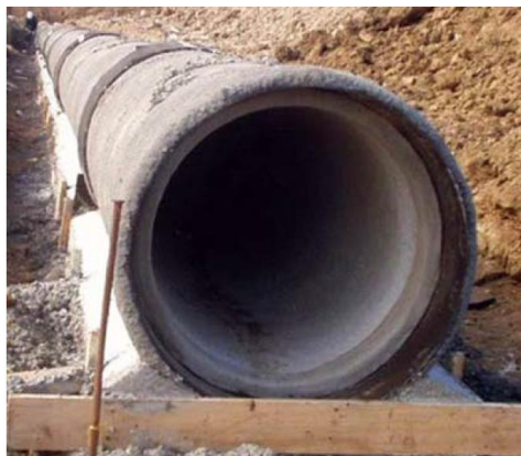
Figure 2. Precast concrete conduit: (a) schematic (b) installation [2]
